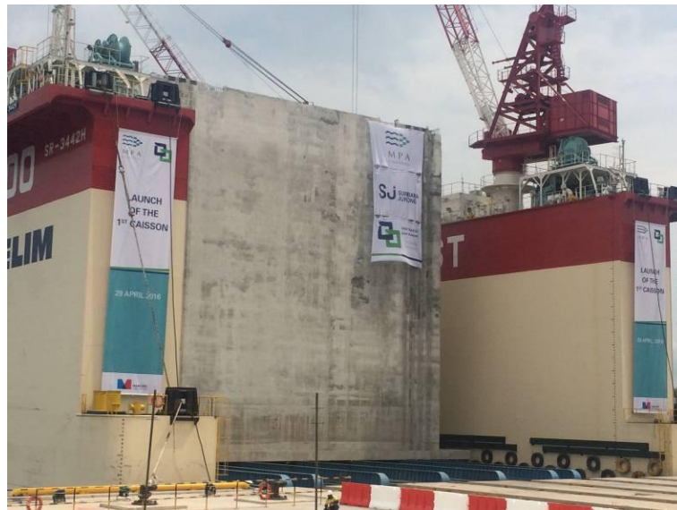
The first caisson transferred onto the floating dock at the Tuas Terminal construction site
