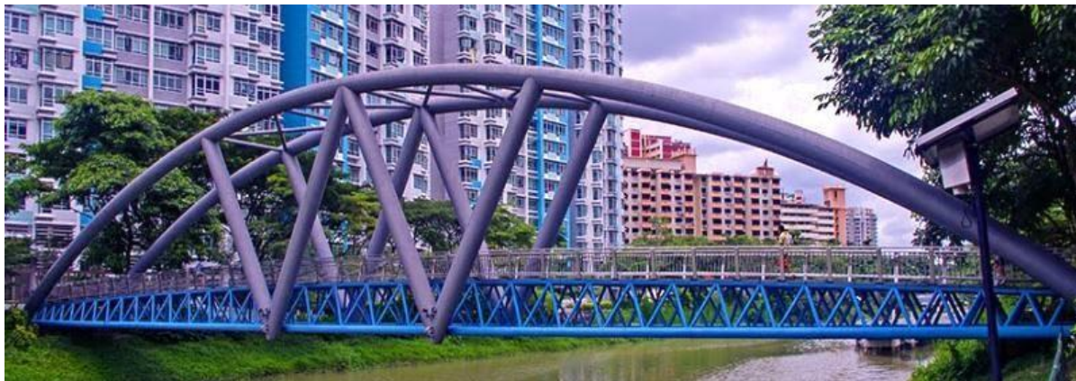
Figure 1.1 A 58m Span Steel Footbridge Across Kallang River, Singapore
