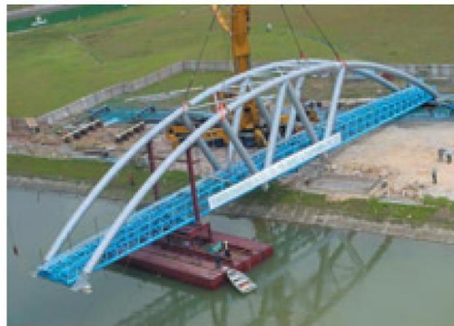
Assembly supported on barge
