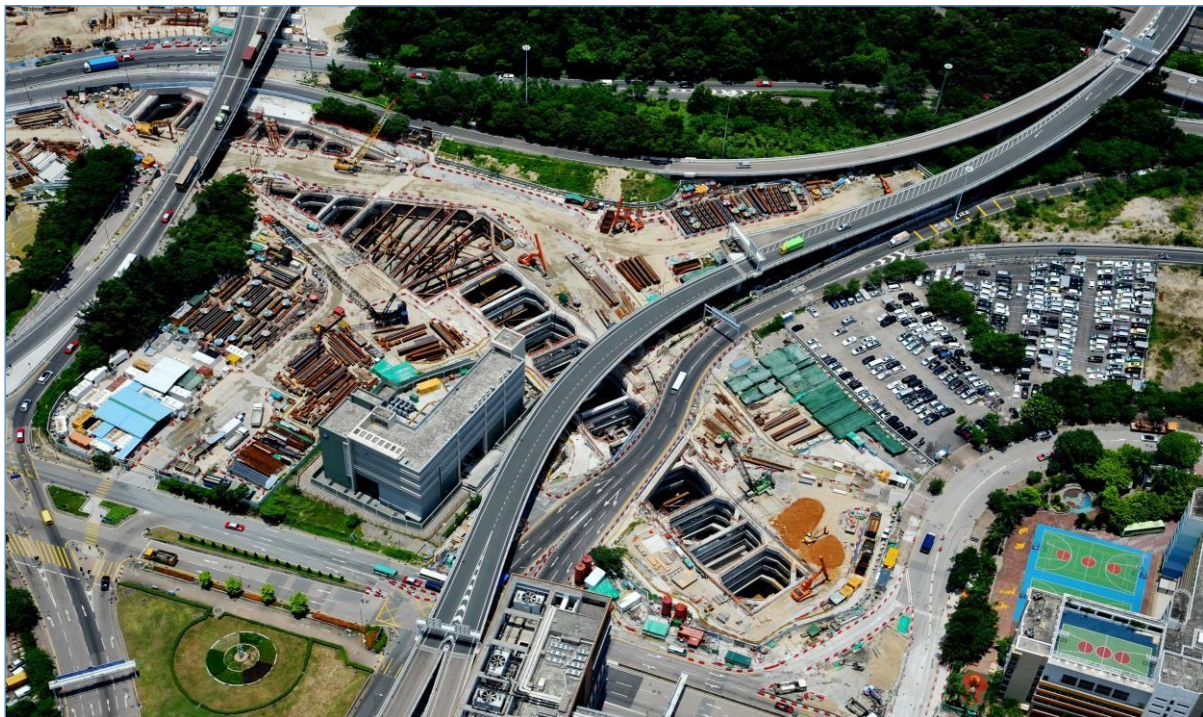
Figure2.2 Aerial Photograph of Construction
