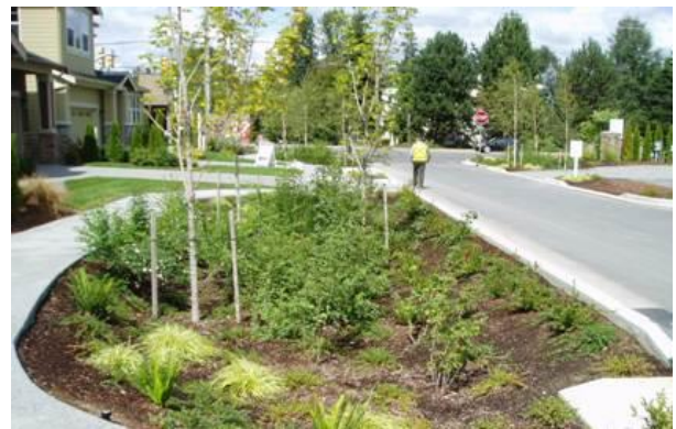
Road Side LID (Source: City of Kirkland)
